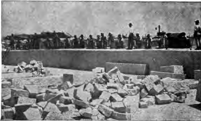
Fig. 136. Splitting Granite by Compressed Air, at Mt. Airy.
